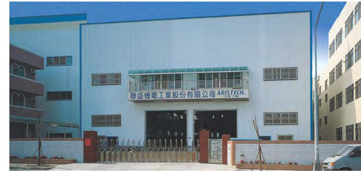
◆ THE NEW SECOND PLANT
